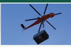
Herman Goldner Co. finished a complete cooling tower replacement in 2018 for Centre Square, the tallest office building in Philadelphia. The building's 40+ year-old wooden cooling towers were past their useful life and leaking, causing an inability to cool the entire building. The project required the use of a helicopter to lift the new cooling towers to the roof. The replacement tower will lead to a reduction in water and energy usage for the building and its tenants.
