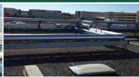
Needing to ensure worker safety and improve its maintenance access to the high pressure steam (HPS) supply for critical buildings at its West Point, Pa., research and manufacturing facility, Merck & Co. contracted Herman Goldner Co., Inc., to work on the installation of new steam mains and isolation valves at seven locations on the campus. The steam is used not only for heating but for research and production processes.
